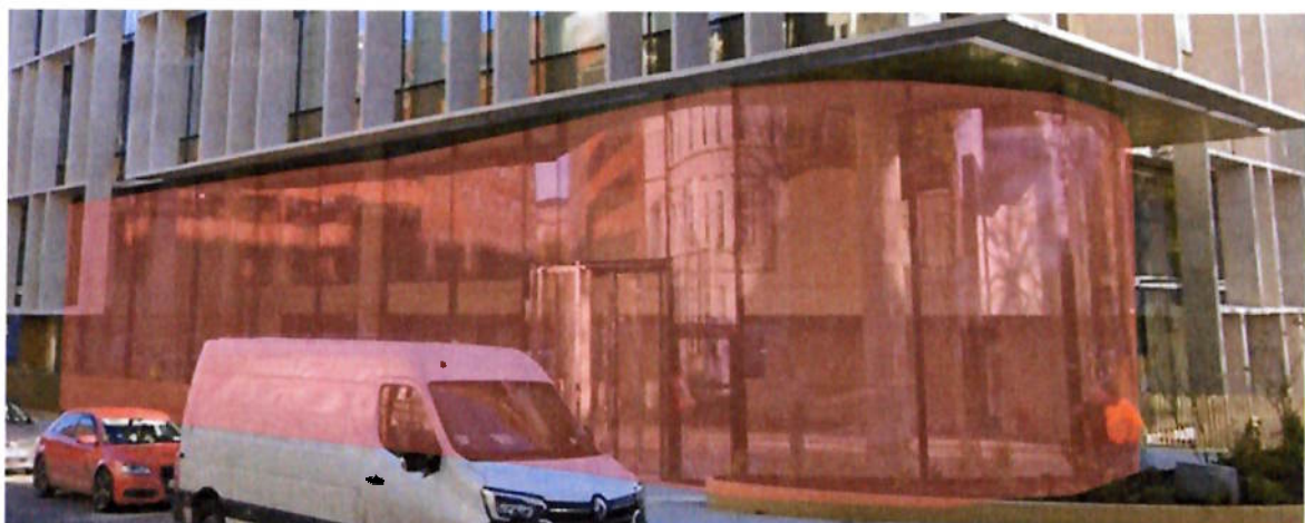
Figure 9 EWS 006 Entrance Glazing elevation scope. 5.7m hespoke curved glass screen
